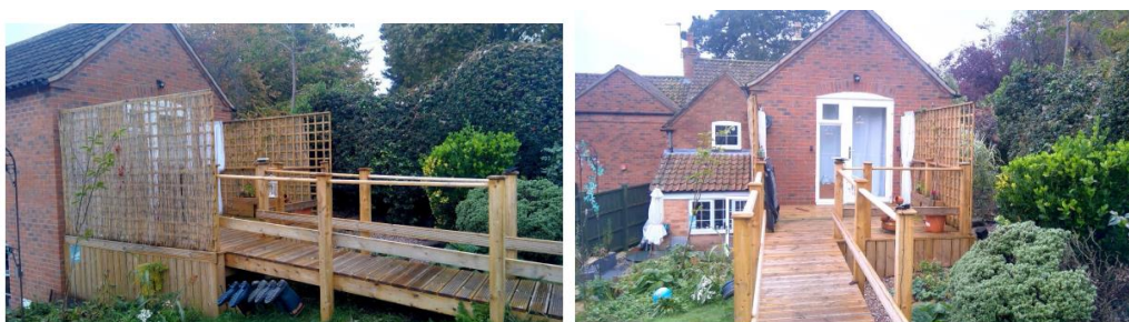
Fig. 5 Site Photos of Development
